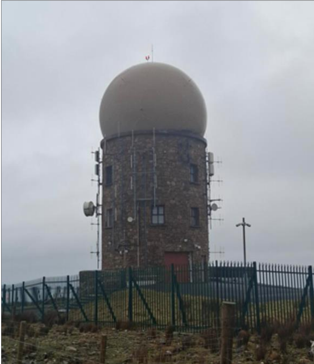
Figure 13. Dooncarton SSR Radar Station
